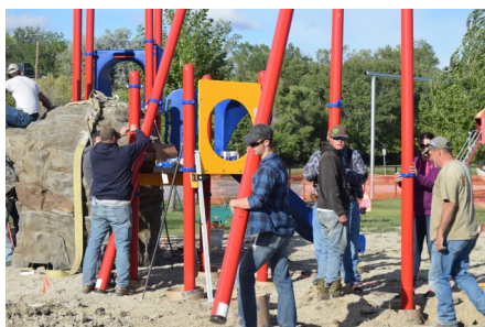
Volunteers installing the new playground equipment at Chief Joseph Park.
